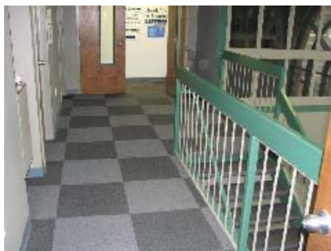
Pictured here, Paraweave soft tile flooring appears in a commercial setting. The checkerboard effect is created by turning the tile so it refracts light from a different angle.
